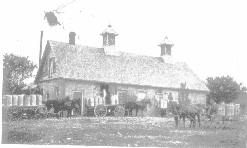
THIS VIEW SHOWS BUILDING FULLY COMPLETED.
