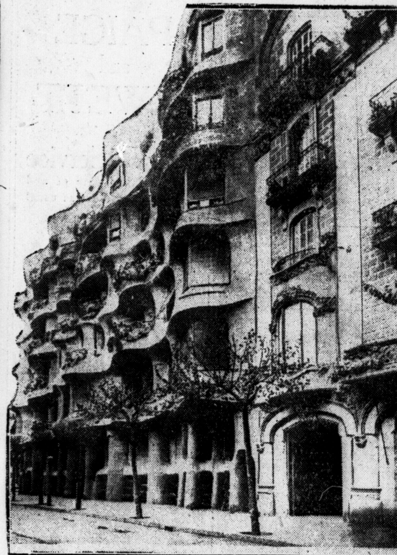
The house of one hundred curves. A unique bit of Spanish architecture in the Catalonian style, which is to be found in Barcelona.
