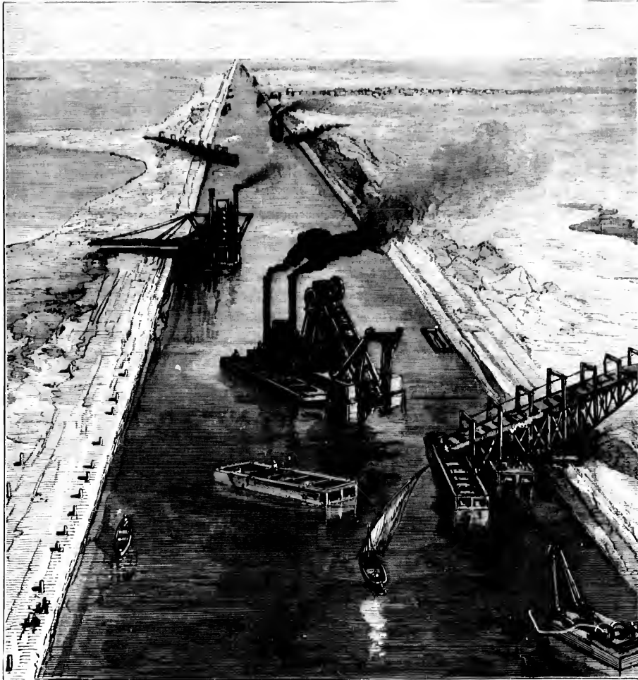
THE SUEZ CANAL: DREDGES AT WORK.
