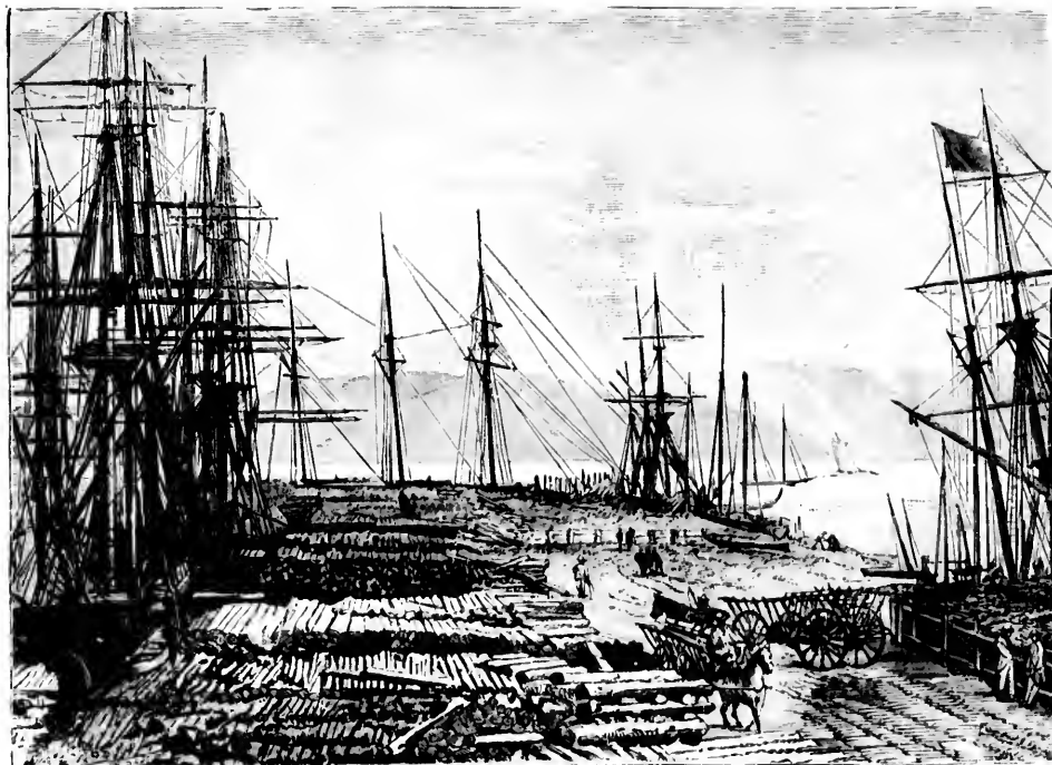
A TIMBER WHARF AT SAN FRANCISCO.
