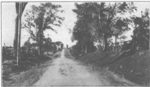
An inexpensive, but serviceable road in Hastings County. It has been gravelled and proper provision made for drainage.
