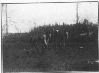
Boring the Holes—Short Work
