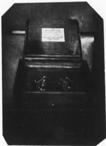
Insulated Tank Containing Cold Water, or Cold Water and Ice, for Cooling Cream.
