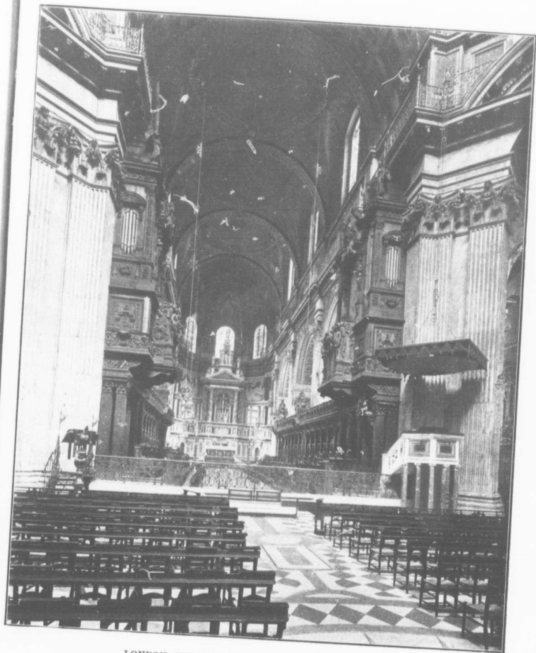
LONDON—INTERIOR VIEW ST. PAUL'S CATHEDRAL.
