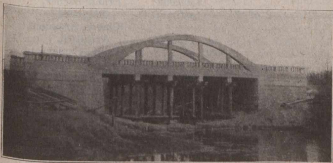
CONCRETE TRUSS BRIDGE AT WILLOW CREEK, MAN.
