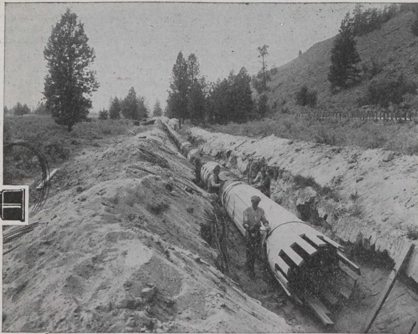
48 in. CONTINUOUS STAVE LINE.
