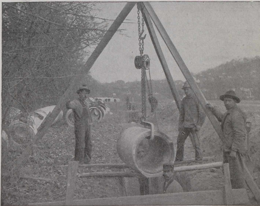
A Triplex Block hung from a temporary rigging and used for laying pipe.
