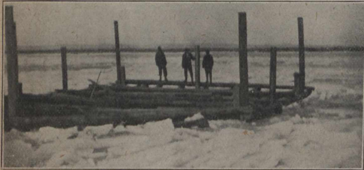
Nose of Protection Pier ready to sink.
