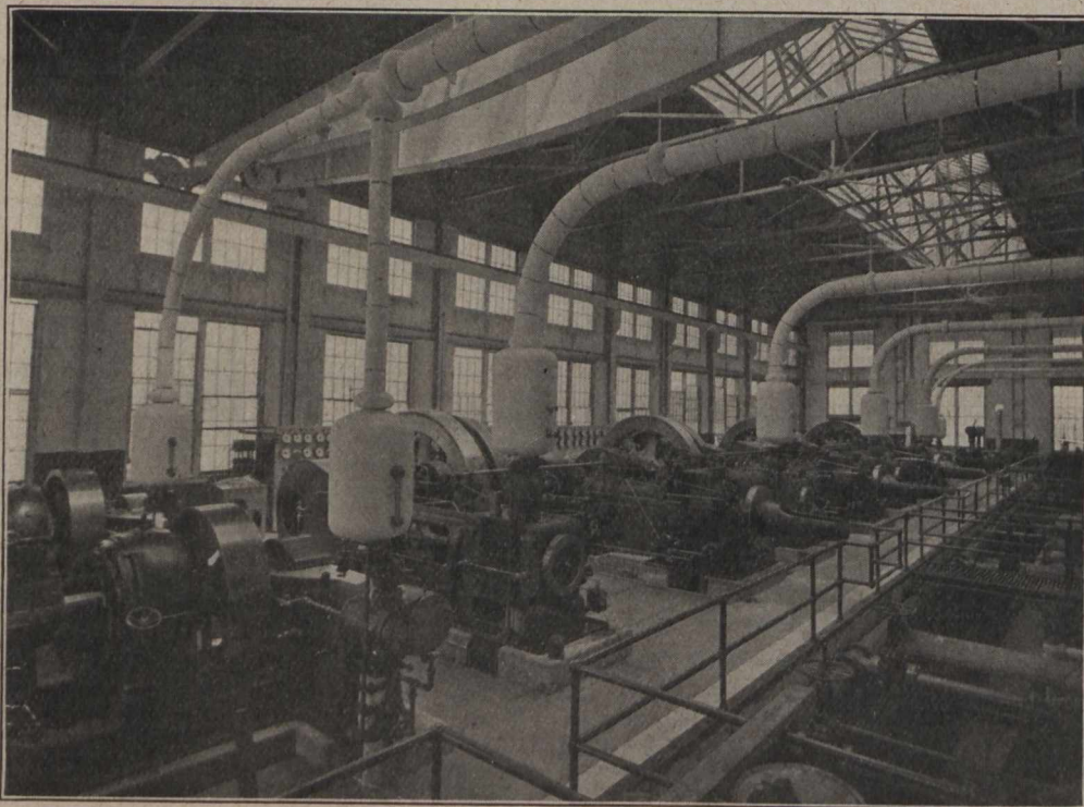
View of Engine Room, from South West Corner.
