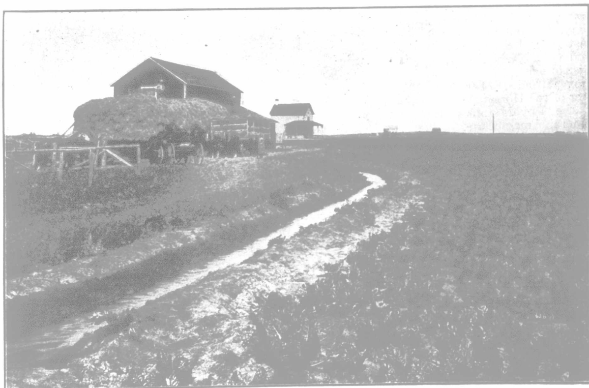
A DISTRIBUTING DITCH ON AN IRRIGATED FARM, ALTA.
