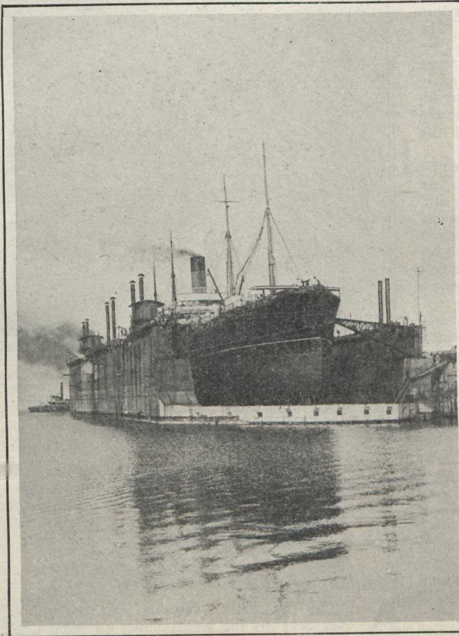
The Canadian Vickers Company carried out their first real job with their floating drydock at Montreal when they repaired s.s. Mount Temple. This picture shows the vessel in the dock, off the Maisonneuve shore.
