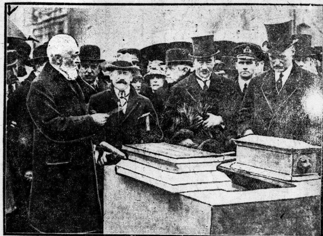
Baron de Bishoven, governor of Western Flanders, unveiling the foundation of the monument to the British navy, which is being erected at Zeebrugge.
