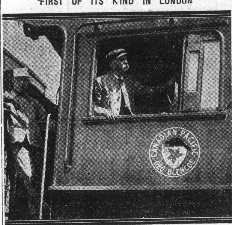
C. P. R. engine now known as "George Blencoe," because of the meritorious record of the engineer who pulls its throttle. This is the first engine to be so named running out of London, although it is the second in the division.
