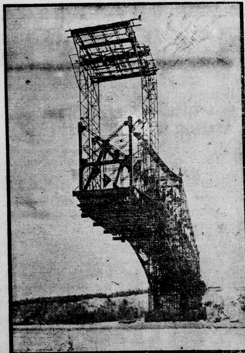
VIEW OF COLLAPSED SECTION OF QUEBEC BRIDGE AS SEEN FROM THE RIVER.
