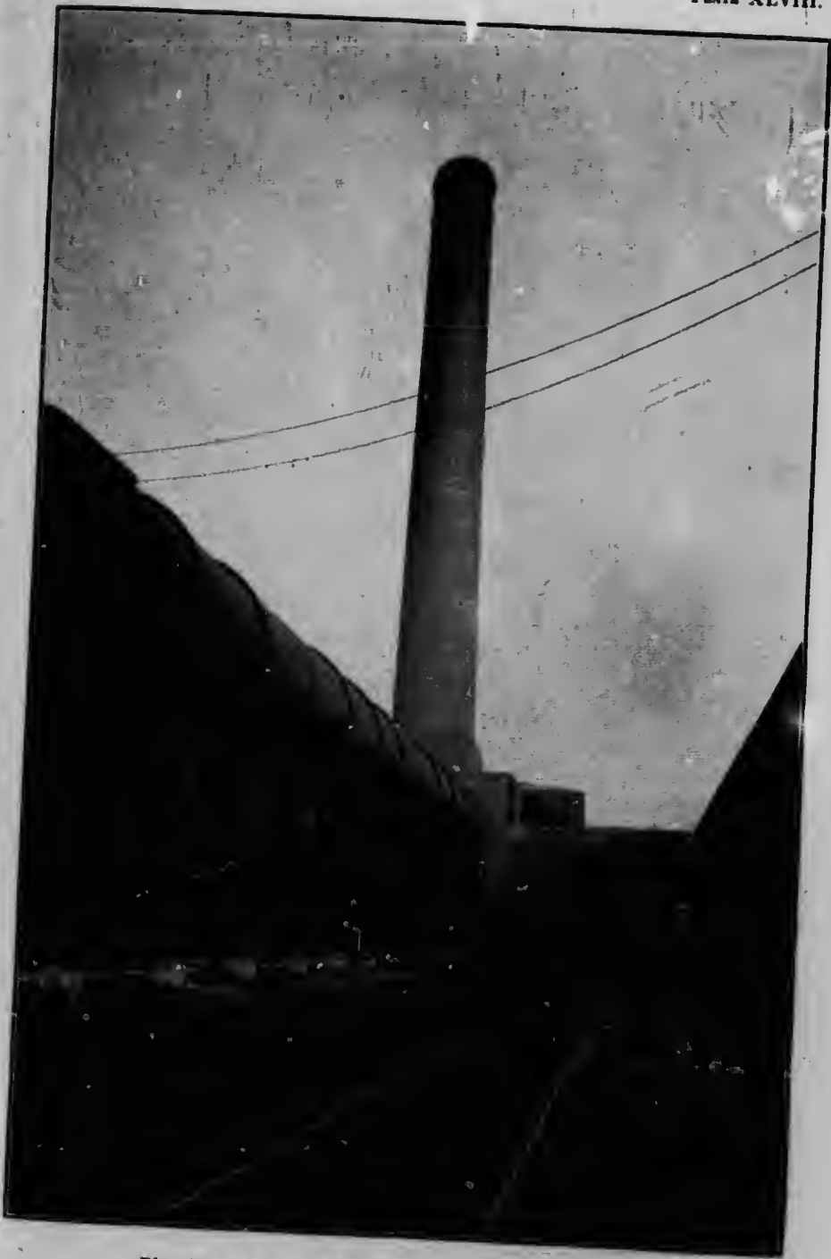
Blast furnace flue: Canadian Copper Co. smelter, Copper Cliff.
