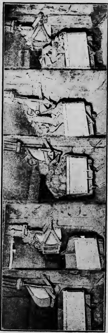
Air-operated chute gates.
