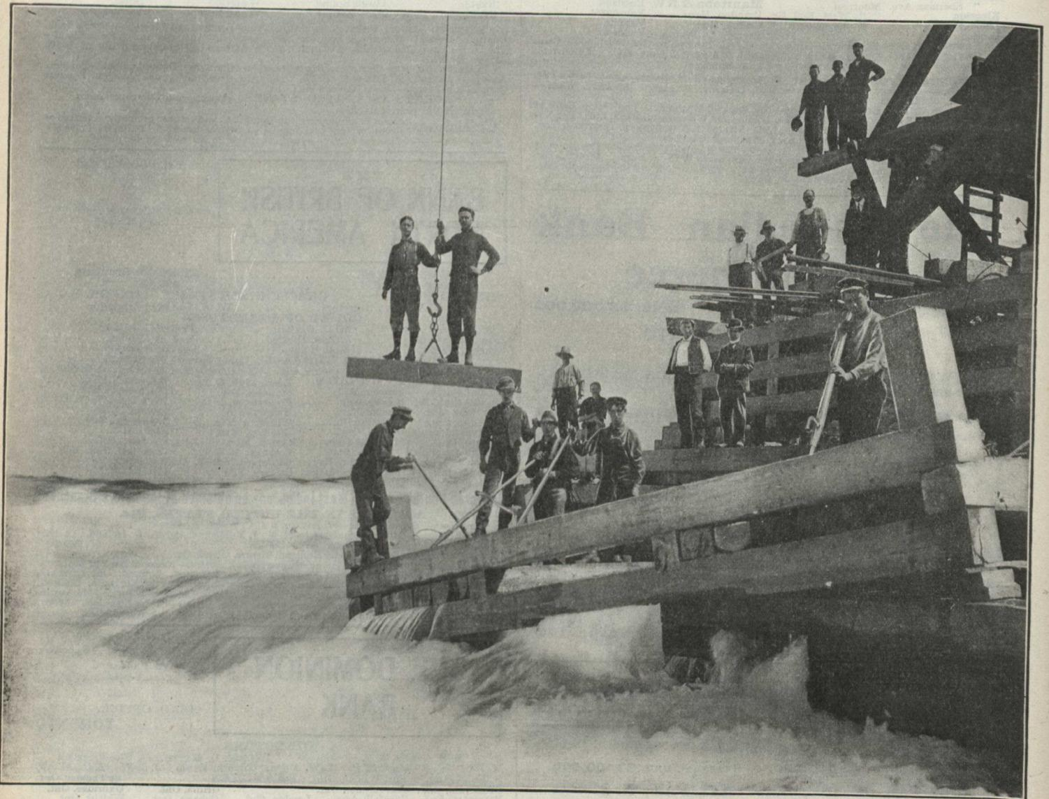
Launching of a Crib in the Cascade Rapids, Niagara River. Works of the Electrical Development Co. of Ontario.
