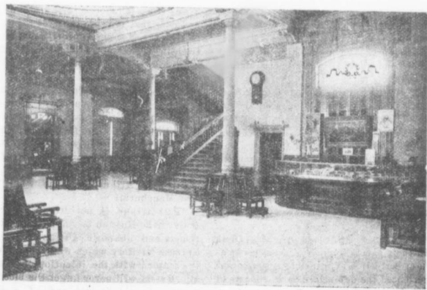
The Russell House, Ottawa—The Rotunda at 5 o'clock in the morning
