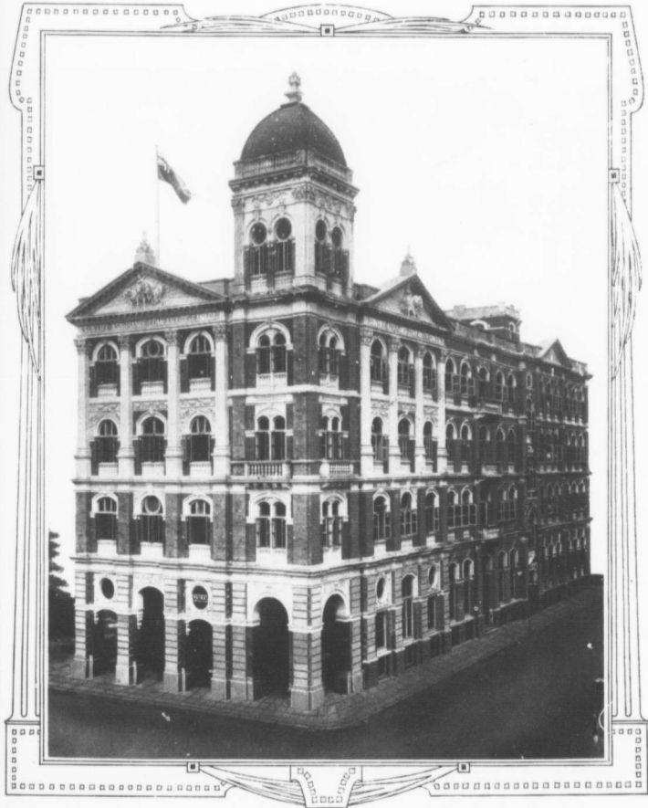
CANADA BUILDING, BOMBAY. Headquarters of the Sun Life Assurance Company of Canada in India.
