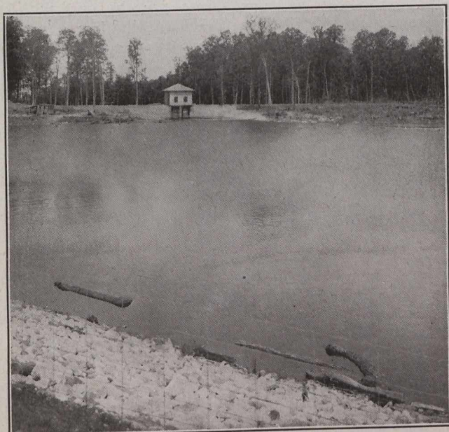
Fig. 7.—Gate House and Forebay, from No. 2 Dam.
