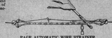
PAGE AUTOMATIC WIRE STRAINER. The best tool made for erecting and repairing wire fences of all kinds.
