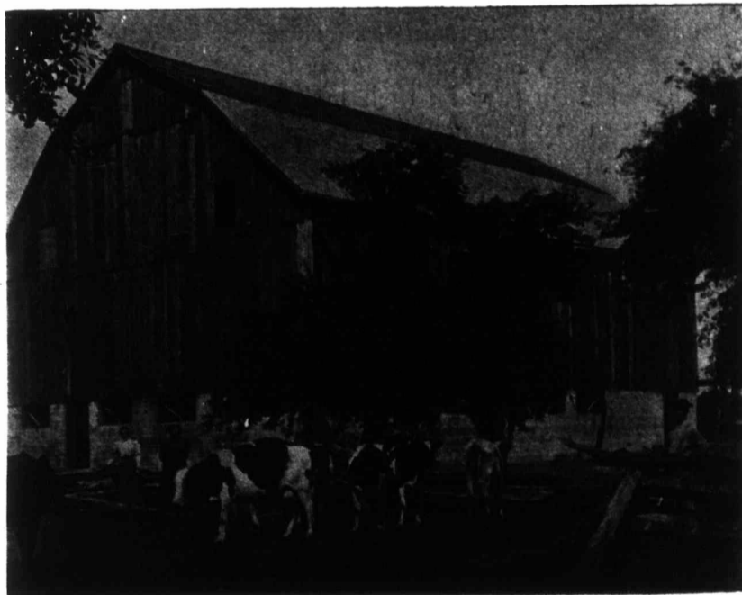
BARN OF THOMAS HARTLEY, NEAR NORWICH, ONT. Size of Basement Walls, 50 feet x 68½ feet x 9½ feet high.
