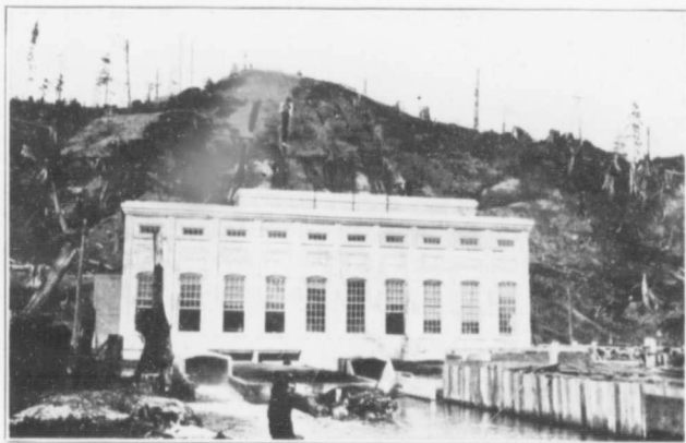
Jordan River Power Plant
