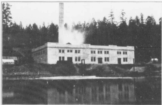
Brentwood Steam Plant
