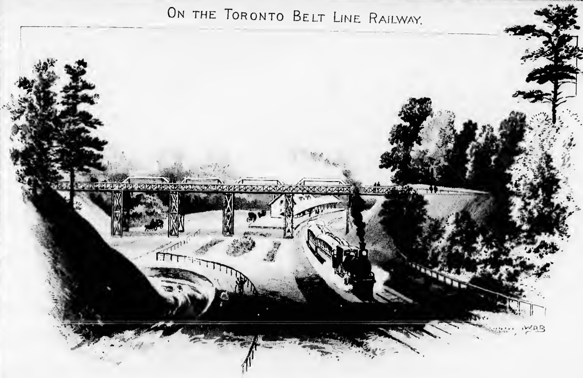
STATION AT MOORE PARK - AND NEW HIGHWAY BRIDGE.
