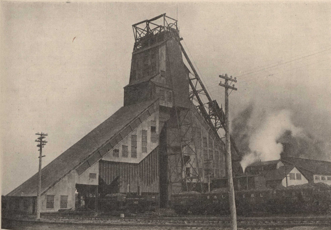
Dominion No. 2 Colliery. Bankhead for Phalen and Harbour Seams.
