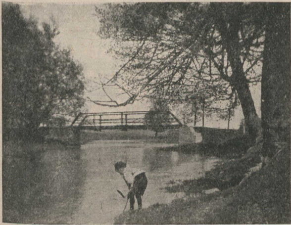
The old Creek and the Bridge—A luring spot to the small boy.
