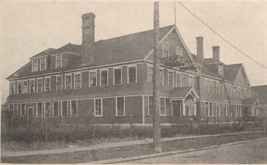
General Offices of the Dominion Coal Company, at Glace Bay. The Employees of the Company are on Strike.
