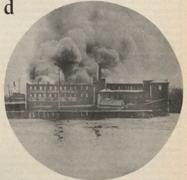
FIRE IN THE MIDST OF WATER. A Flooded Planing Mill on Fire in Columbus.
