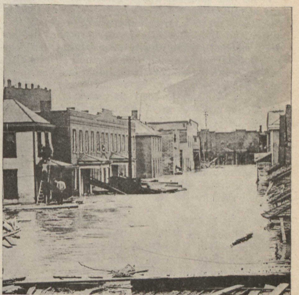
WHERE SHOPS CLOSED UP. Business Street in Dayton Completely Under Water.
