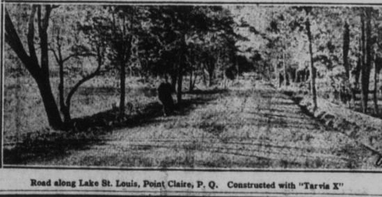
Road along Lake St. Louis, Point Claire, P. Q. Constructed with "Tarvia X"
