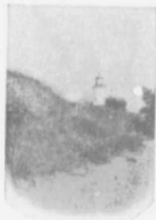
BOIS BLANC LIGHTHOUSE ERECTED IN 1828
