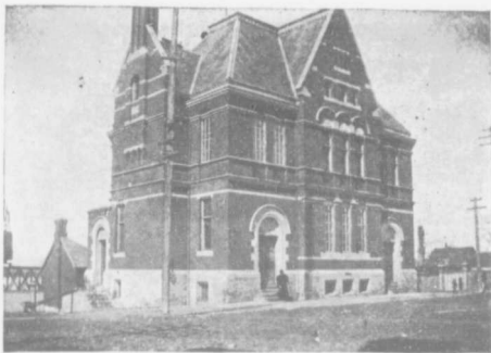
DOMINION GOVERNMENT BUILDING.
