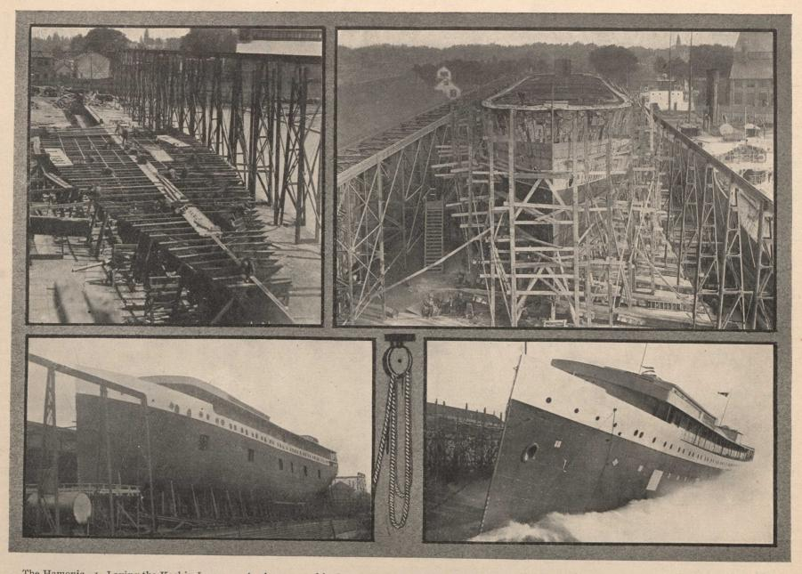
The Hamonic—1. Laying the Keel in June. 2. As she appeared in September when the third deck was reached. 3. Ready for Launching, with part of the Aerial Railway taken down for this purpose. 4. As she slid into the water of the Dry-Dock.
