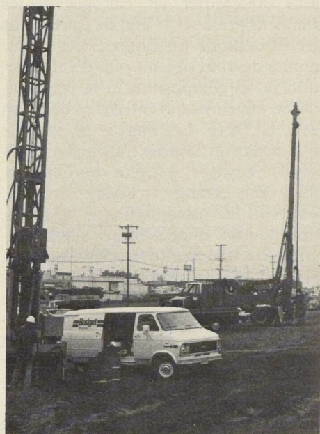
Drilling for soil samples on the Regina factory site reached depths of 27 m to evaluate pollutant migration. (Photo: J.R. Roberts, Div. of Biological Sciences)
