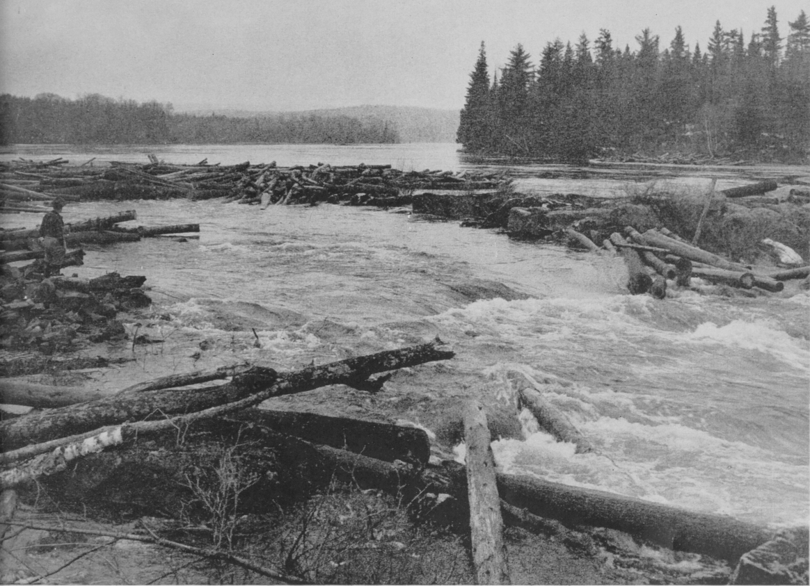
Looking upstream prior to construction of Des Joachims Dam—from Ontario side.
