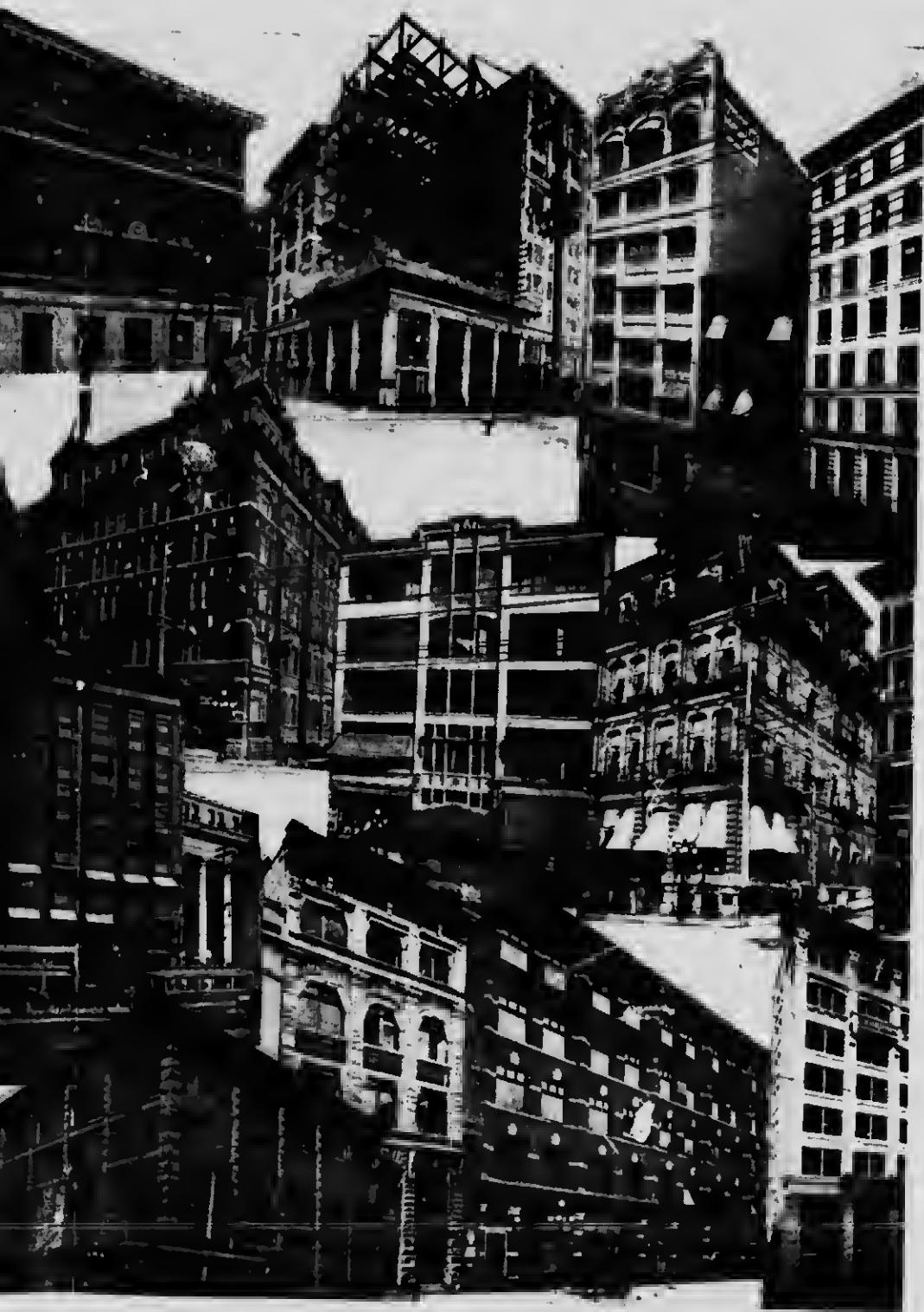
No Place in Canada is Building Better than the Capital City.
