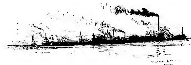
CEMENT WORKS, NORTHFLEET HOPE.
