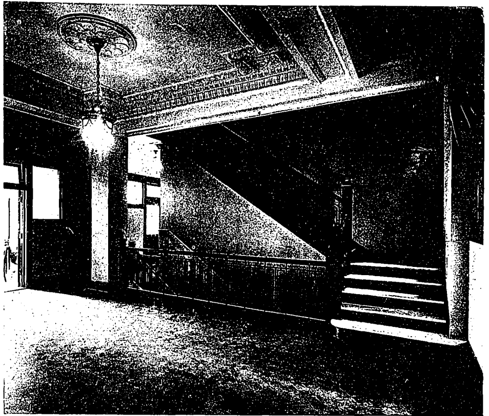
UPPER HALLWAY, HYDRO-ELECTRIC BUILDING, TORONTO.
