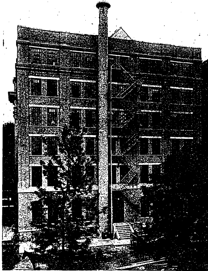
REAR VIEW, HYDRO-ELECTRIC BUILDING, TORONTO. E. T. BRANDON, ARCHITECT AND ENGINEER. GEO. W. GOUINLOCK, CONSULTING ARCHITECT.
