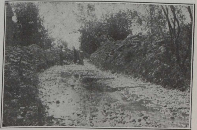
Mountain Lake, Approach Channel to Weir.
