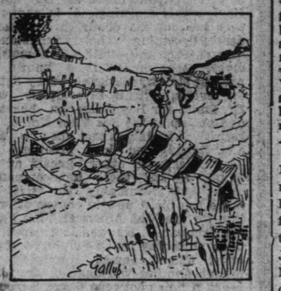
Built shortly after the War of 1812, and affected by the weather to quite an extent.
