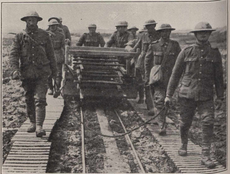
Light railway laid over captured ground on the British Western Front. Official photograph issued on behalf of the Press Bureau. Crown copyright reserved.
