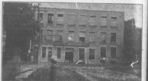
The Fine Plant of "The Guelph Creamery Company," Guelph, Ont.
