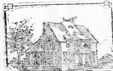
REAR VIEW OF COUNTRY RESIDENCE.
