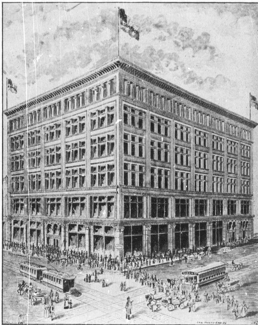
R. SIMPSON'S MODERN DEPARTMENTAL STORE, S. W. COR. YONGE AND QUEEN STS., IN COURSE OF ERECTION.
