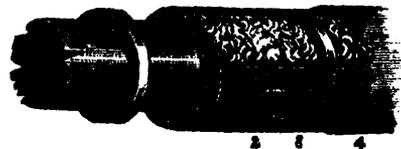
Fig. 4.—Mineral Wool within Wooden Collars, made in Sections and Protected next to the Pipes by Tin or Sheet Iron.
