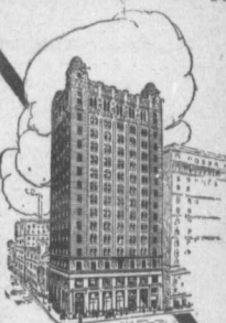
C.P.R.'s Great Offices in Toronto. Roofed with Natco Hollow Tile.
