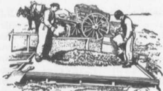
THE mixing and placing of concrete is simple, and is easily learned. No elaborate tools are needed.
