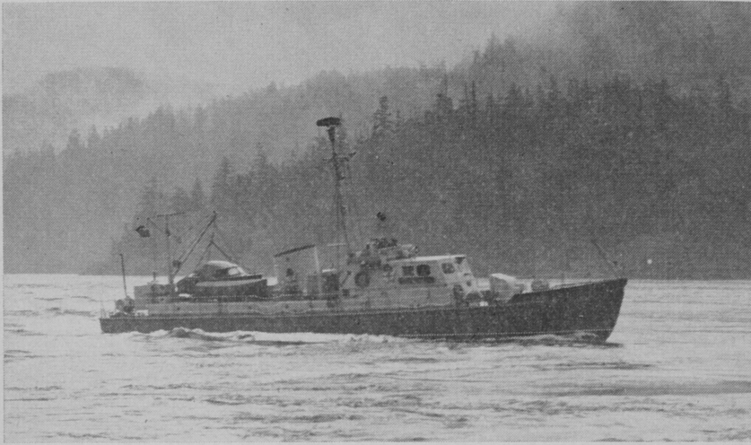
Approximately 10 a.m., April 5. The RCMP Victoria flying the Lieutenant-Governor's pennant, steams over Ripple Rock, the first ship to pass through after the blast.
