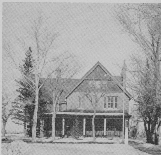
Officers' Mess, Regina, Sask., prior to commencement of demolition.
