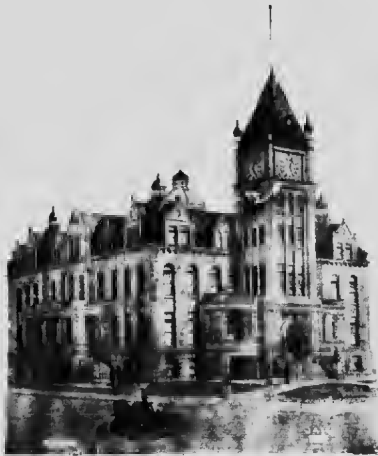
VIEW OF CALGARY'S NEW CITY HALL.
