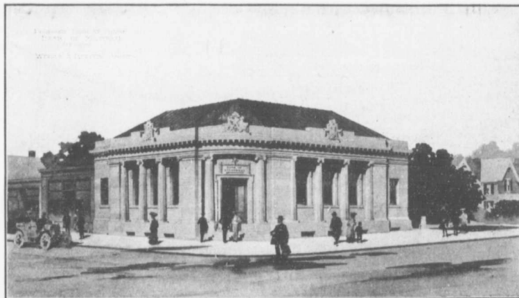
BANK OF MONTREAL, BANK STREET BRANCH.
