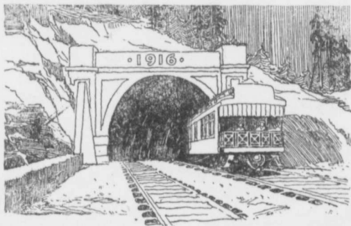
East portal, Connaught Tunnel
