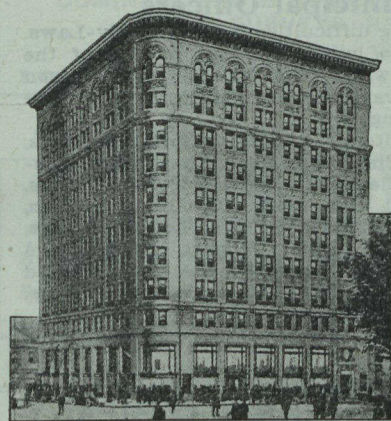
Birks Building Vancouver, B.C.
