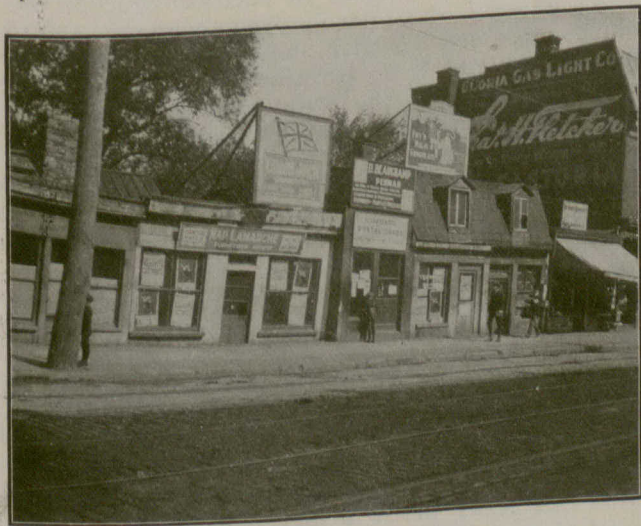
Many changes in St. Catherine street are promised for the near future, but the only large work at present in progress is the Lindsay Building on the south side of the street a little west of Peel street. There is little of this showing as yet but the work has
