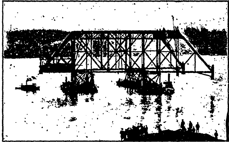
Floating the spread span into position on scows.
