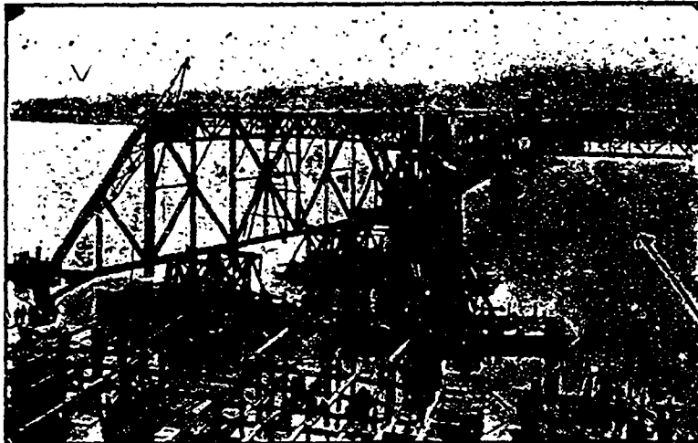
General view of the structure just after the spread span had been floated into place on its piers.
