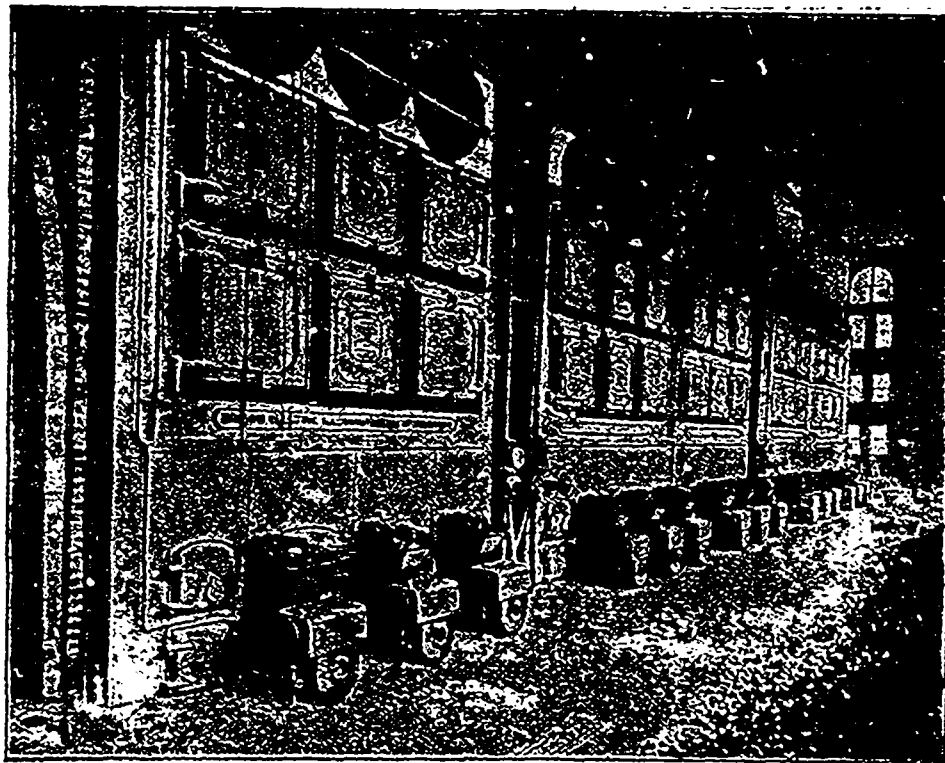
PLANT EQUIPPED BY THE AMERICAN STOKER CO., SHOWING THE AUTOMATIC STOKERS, AS IN USE AT UNION STATION, EDISON ELECTRIC ILLUMINATING CO., BROOKLYN, N.Y.
